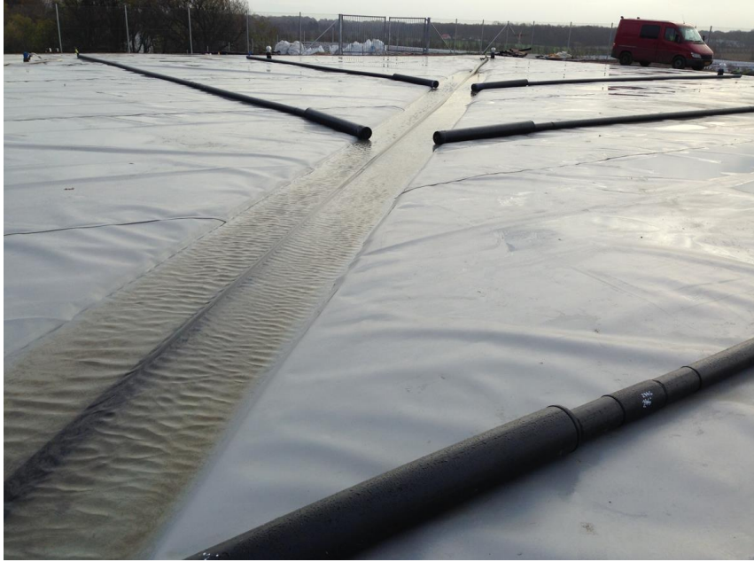
Figure 12. Foto from Dronninglund Lid Design with black HDPE pipes
