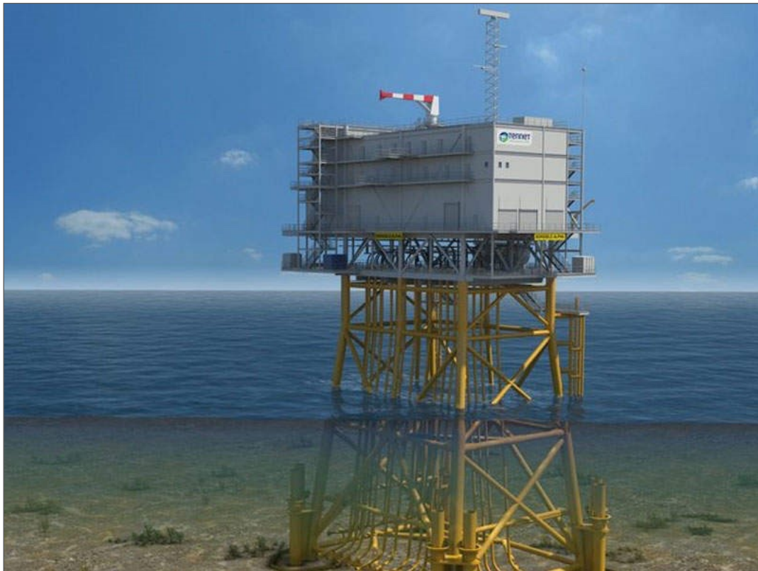
Figure 5 Jacket structure showing complex geometry and obstructions
