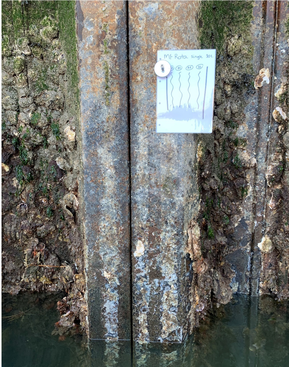
Figure 11 Well performing water jet nozzle after four runs.
