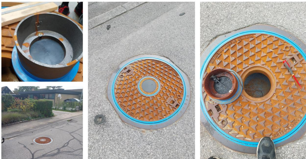
Figure 3 Special lids with integrated composite material investigated by Kredsløb for data transmission above the ground.
