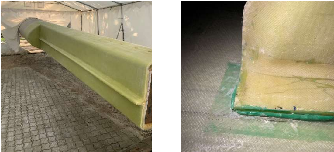
Figure 17: Repaired blade section (on the left) and initiated crack in the aft shear web bondline (on the right).
