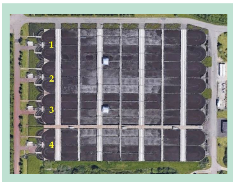
FIGURE 23. Overview of the biological nitrogen removal (BNR) at Avedøre wastewater treatment plant show four biological lines each consisting of two process tanks. (Background image: Google Maps, Image © 2022).
