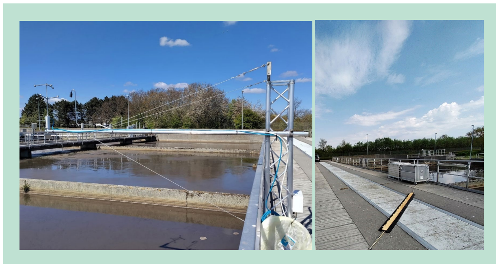
FIGURE 17. Description of the EC system. Photos of the EC mast with the ultrasonic anemometer and the gas inlet above the aeration tanks (left panel) and the containers housing the closed-path \text{N}_2\text{O}/\text{CO}/\text{H}_2\text{O} analyser and the vacuum pump (right panel).
