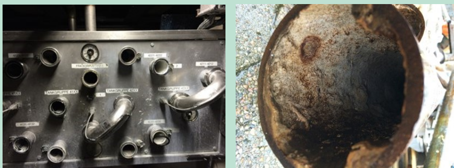
Figure 25. Pipe Connection point for connecting different tanks (left). Discarded production pipe with paint residues (right).
