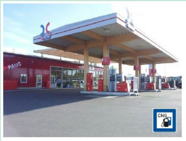
BILLEDE 3 LNG/CNG TANKSTATION (LIQUILINE)
