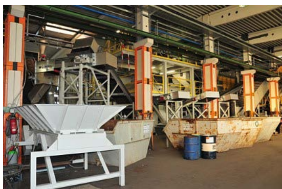
Figure 3.9 A view inside the WEEE treatment plant Adamec (Lang 2011)
