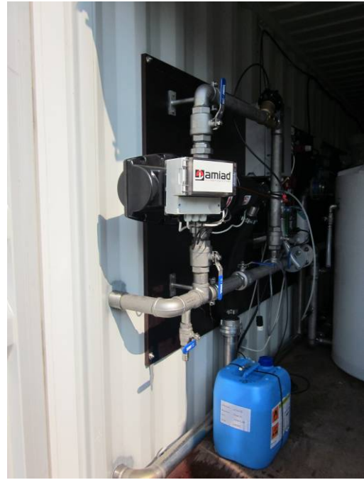
Fig. 7: Amiad pre-filter + biocide dosing
