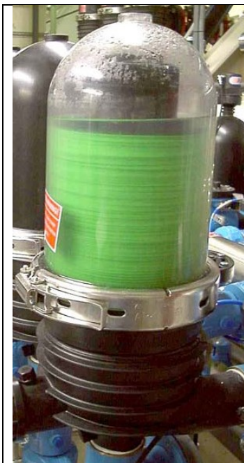
Figure 12. Disk filtration (Picture: Hyde Guardian using disk from Arkal filtration systems. (Source: hydmarine.com )
