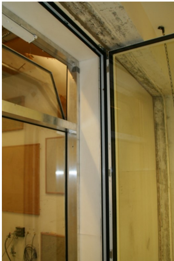
Figur 36: Indsat karmabsorbent.
