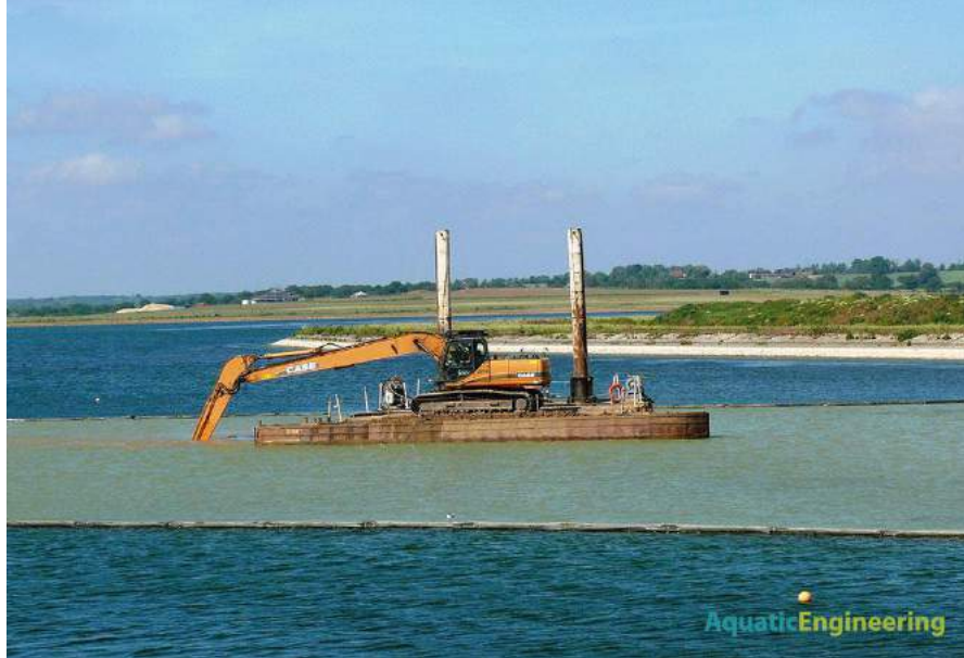
Figure 8 Example of silt curtain from (“Aquaticengineering,” 2022)
